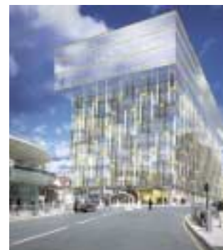
Palestra, SE1: Construction finally starts
