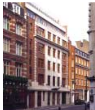
48 Warwick Street, W1: Almost fully let after 4 years of vacancy
