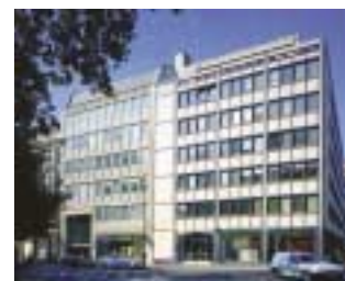
19 Hanover Square, W1: Hammerson commences construction
