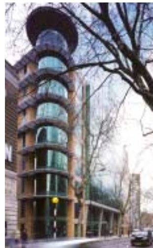
151 Shaftesbury Avenue, WC2: British Horseracing Board deal
