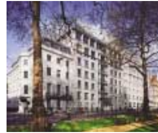
40 Berkeley Square, W1: Deals achieved at £80 psf
